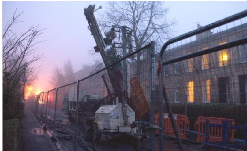
This scheme was carried out for Glasgow City Council and involved treatment of shallow coal workings beneath 3 large residential housing terraces in the Strathbungo Conservation Area. The scheme was secured on a combined Quality/Price tender submission with specific emphasis on proposed methods of work, programme, public relations and management of environmental risks.
