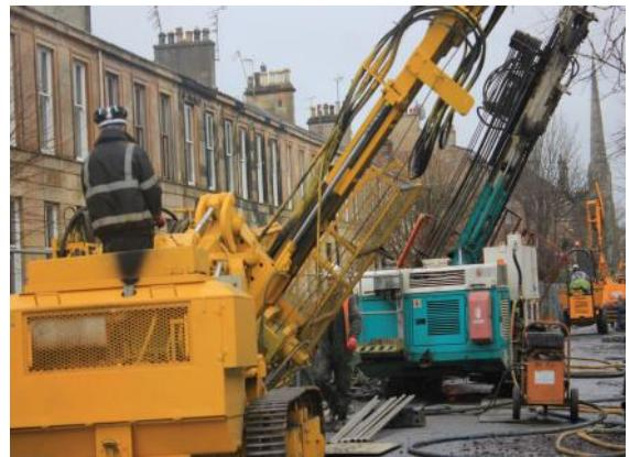
Drilling work was carried out from the streets surrounding the blocks using versatile Casagrande C6 rotary percussive drilling rigs with multi-angling kinematics and smaller Halco 450 rigs which were used in the more restricted back gardens areas.
